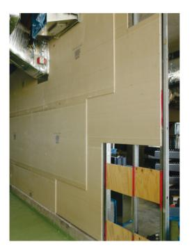
Easy to Cut & Fix: FIBEROCK® AT AR Panels can be cut to size by score and snap process using a paper cutting knife.
